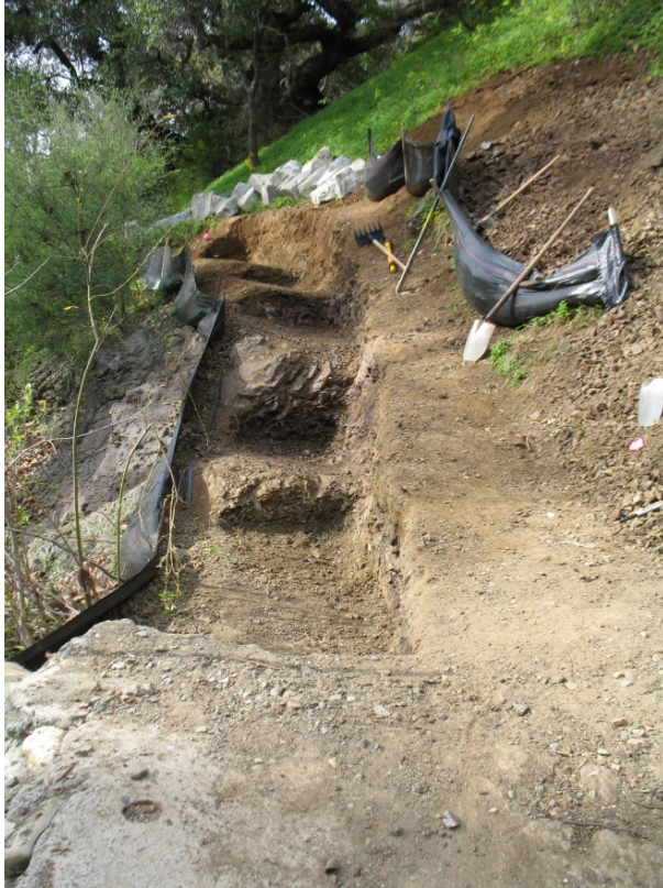
Photo 13.10 - Foundations at Different Elevations
