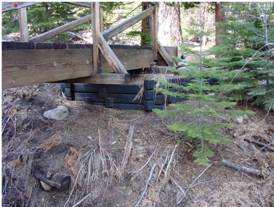
Photo 13.6 - Cribbed Abutment (Using Plastic Lumber)
