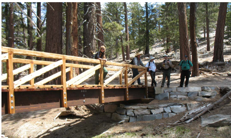
Photo 13.13 - Multi-Tier Rock Approach Ramp
