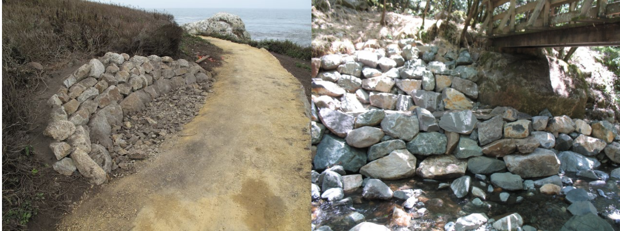
Photo 13.1 - Non-Structural Rock Retaining Walls
