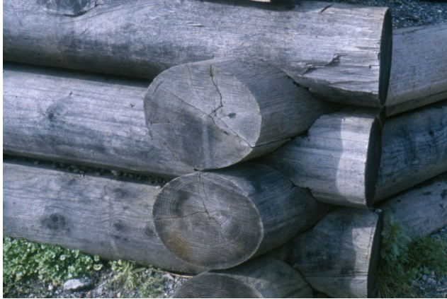
Photo 13.5 - Interlocking Log Walls
