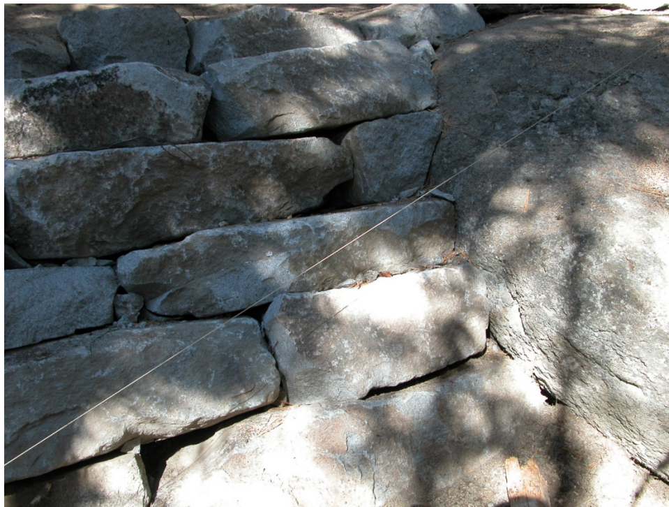
Photo 13.11 - Rock Wall Bedrock Buttress
