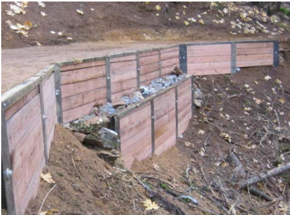
Photo 13.15 - Soldier Pile Retaining Wall
