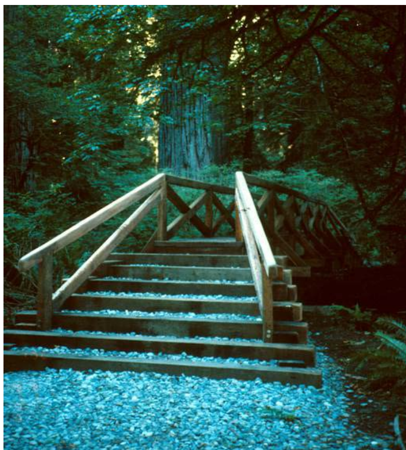
Photo 13.7 – Steps Constructed into a Wooden Cribbed Abutment
