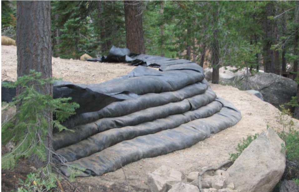
Photo 13.16 - Geotextile Encapsulated Wall
