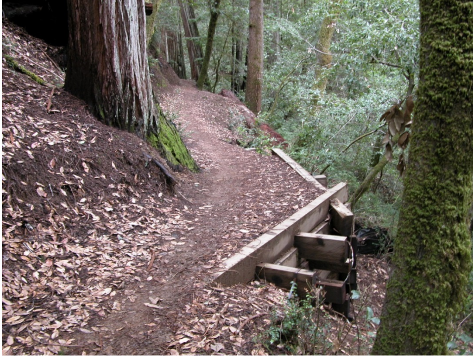
Photo 13.4 - Multi-Tier Interlocking Wooden Structure
