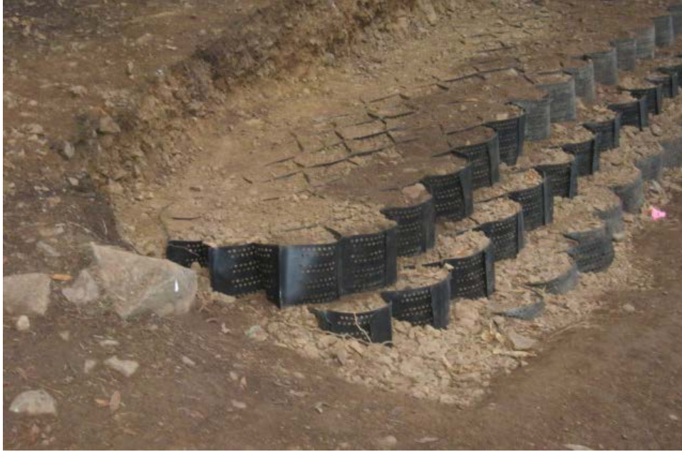
Photo 13.17 - Cellular Confinement Wall
