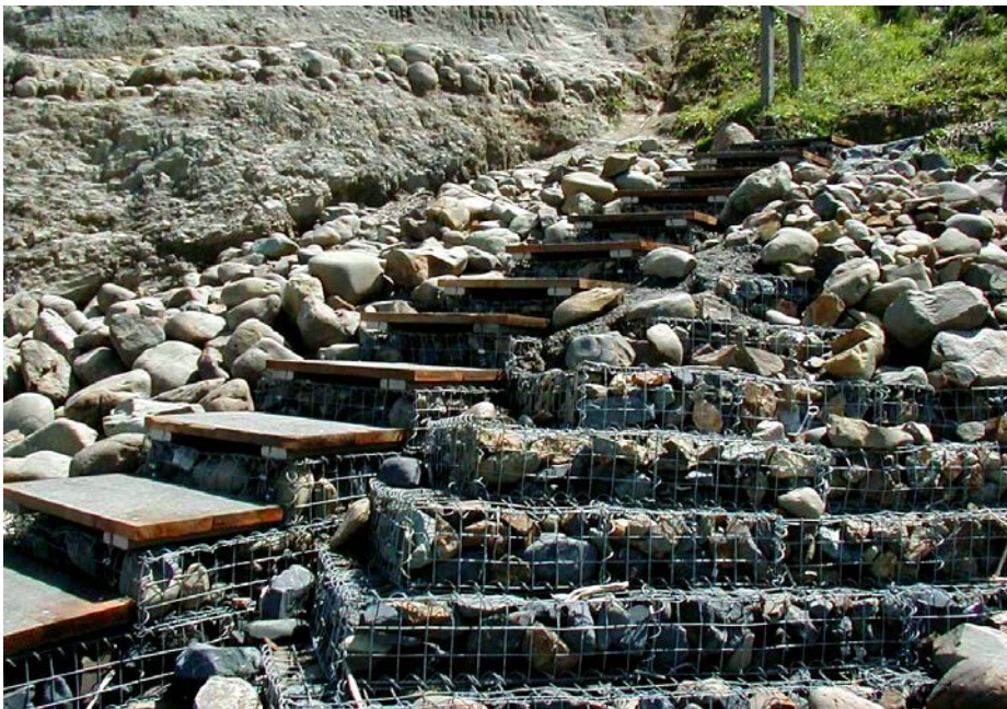
Photo 13.19 - Gabion Walls Prior to Completion of Rock Covering
