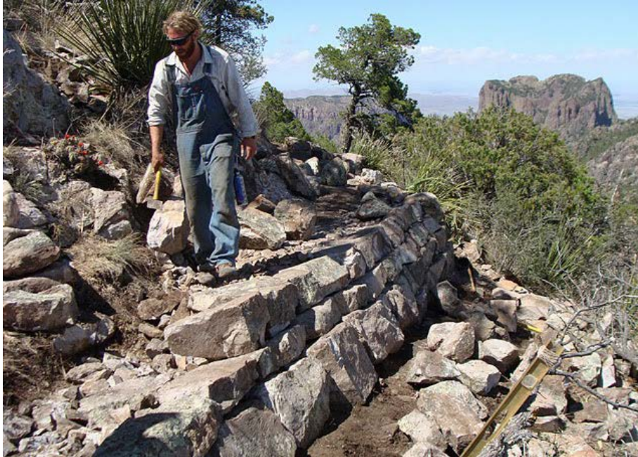
Photo 13.9 - Multi-Tier Rock Retaining Wall
