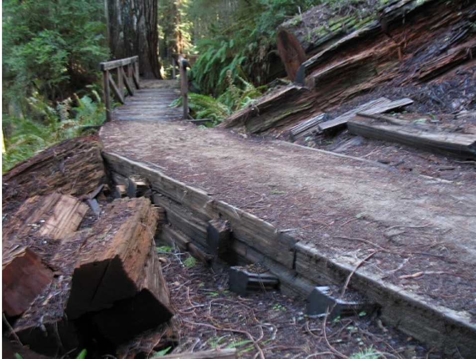
Photo 13.8 - Wooden Cribbed Approach Ramp
